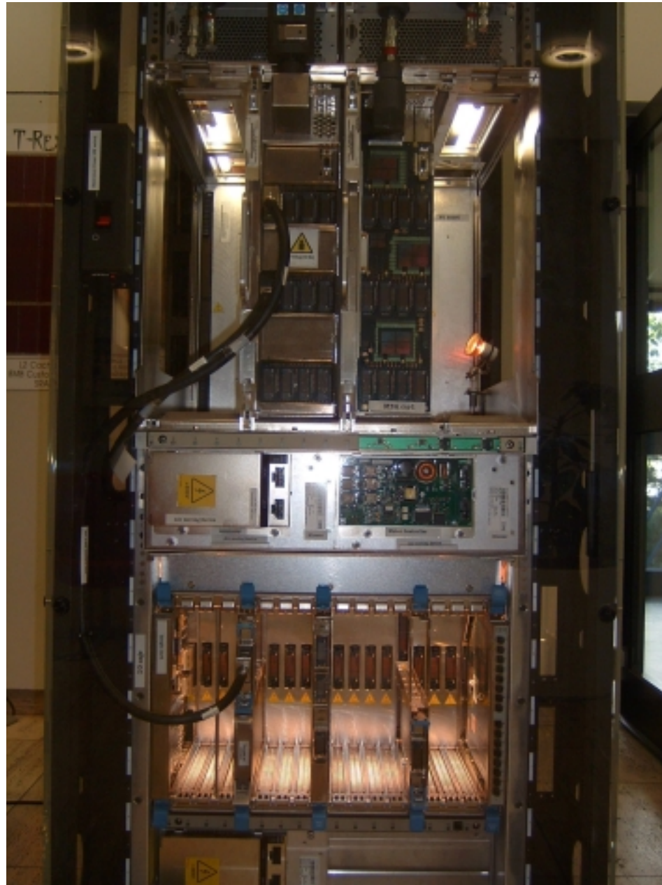
STI cable connection ton an I/O cage
